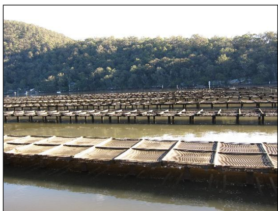
Figure 5. Intertidal trays on post & rail infrastructure.
